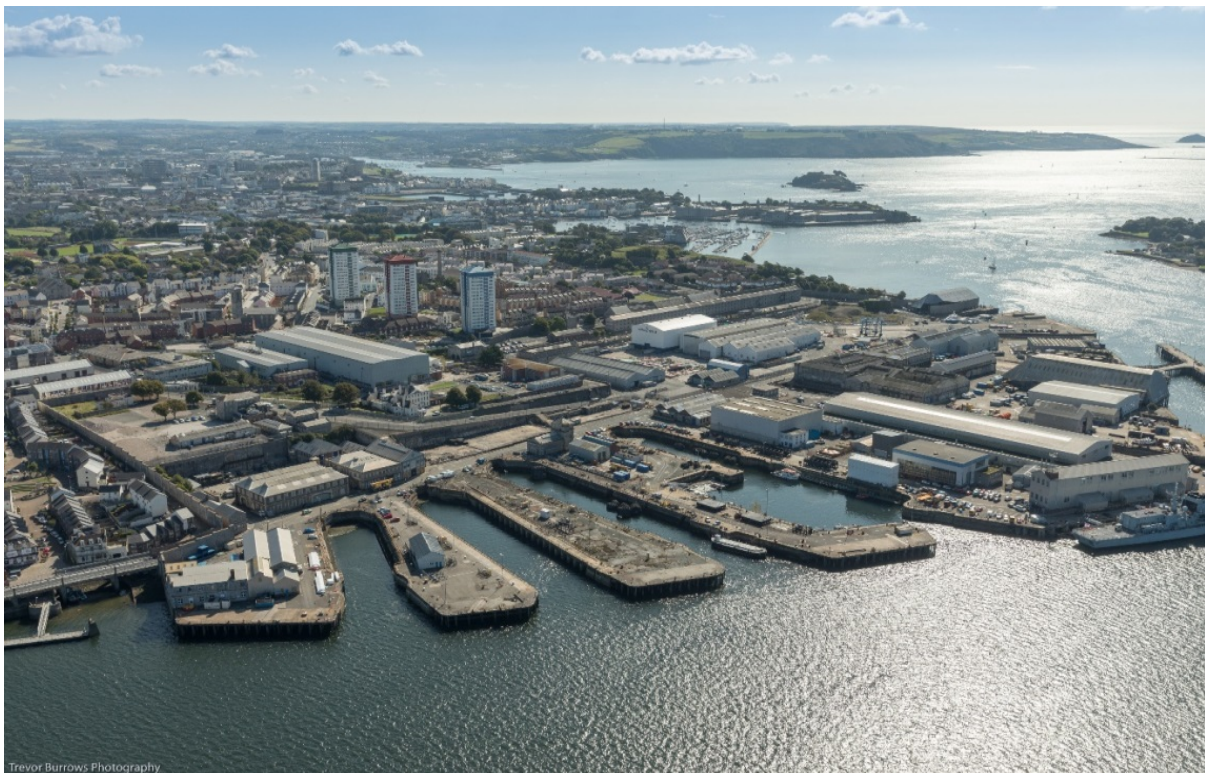
Figure 4 Phase 3 including three docks and associated buildings
